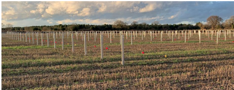
Photo 15.13: Framework Posts being Installed (taken at Tiln Farm, Retford, in January 2023)
