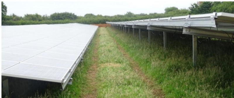
Photo 15.14: Example of Minimal Ground Disturbance Following Panel Assembly
