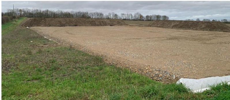
Photo 15.15: Newly Installed Construction Compound
