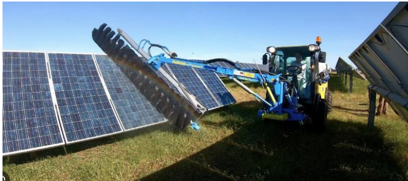
Photo 15.20: Cleaning of Solar Modules
